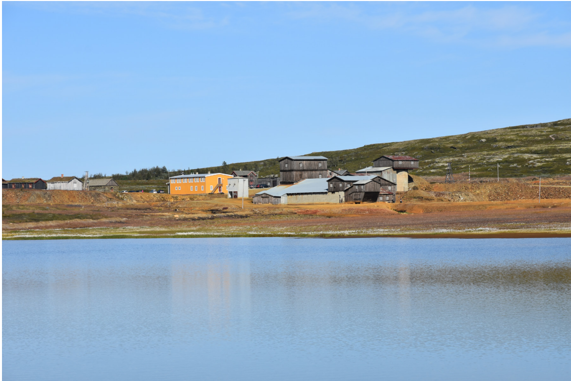
Figure 2. Floatation plant at Nedre Storvartz in Røros Mining Town and the Circumference (Norway). The copper ore from Olav's mine was transported by the overhead cable system. (Source: Author's Photo)
