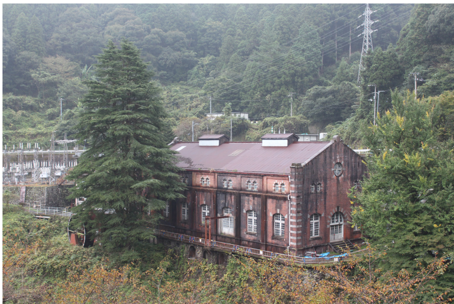
Figure 4. The Hadeba Hydroelectric Power Plant, built in 1912, contributed to the industrialization of the Besshi Copper Mines with its large elevation difference (one of the greatest in East Asia at the time). It also boasted cutting-edge generators and water wheels imported from Germany. The power plant is expected to open to visitors as an educational site in 2022, after the completion of its seismic rehabilitation project.
