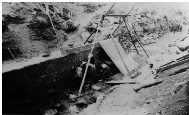
Figure 2. Construction of the trapezoidal weir of the Er-Feng Irrigation Canal System; photo taken between 1922 and 1923 (Photo Credit: Taiwan Sugar Corporation).
