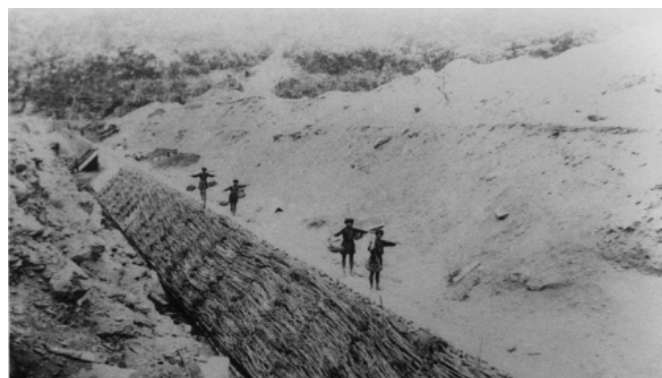
Figure 3. Layers of Simpleleaf Chastetree branches on top of the weir for water filtration; photo taken between 1922 and 1923 (Photo Credit: Taiwan Sugar Corporation).
